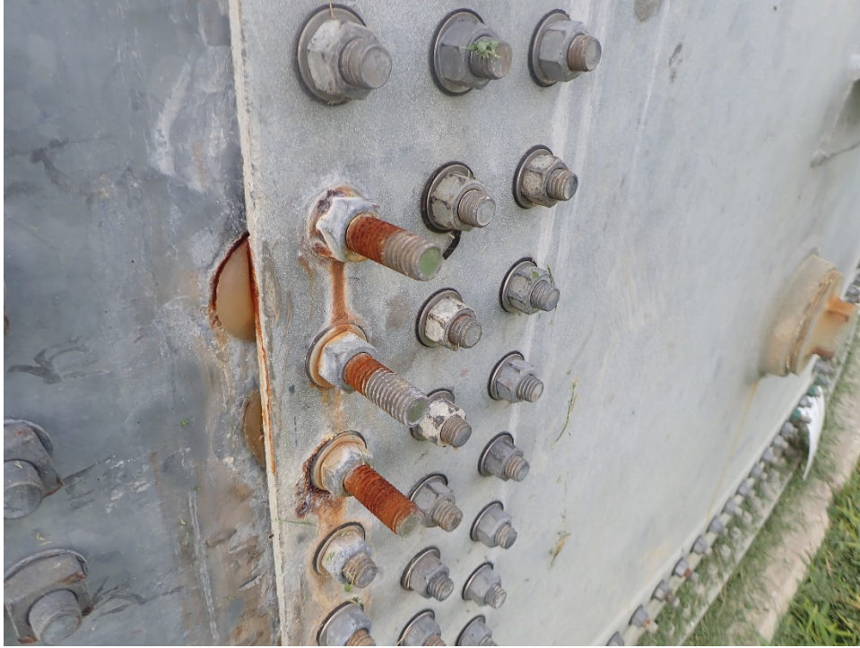
Photo 3: Side hatch with corrosion
