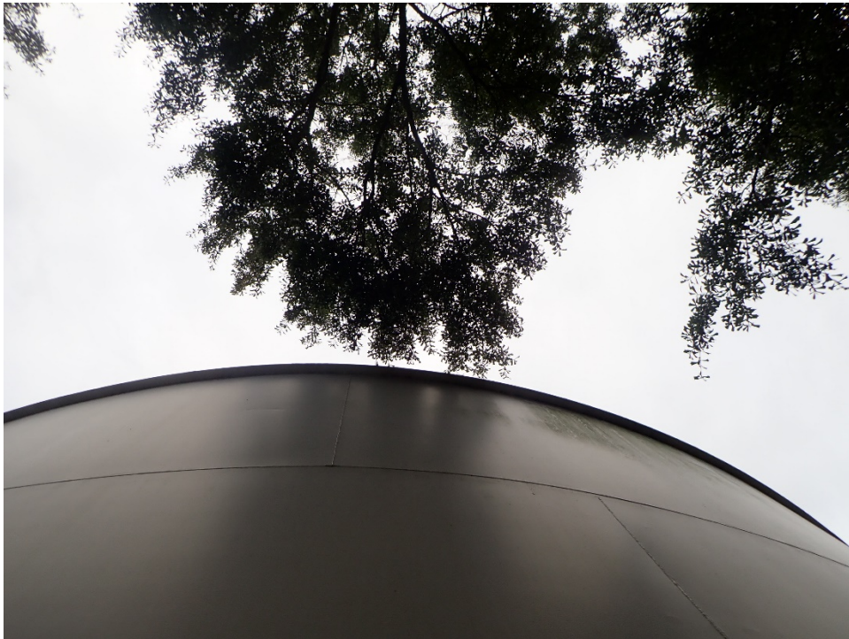
Photo 2: Tank with trees encroaching
