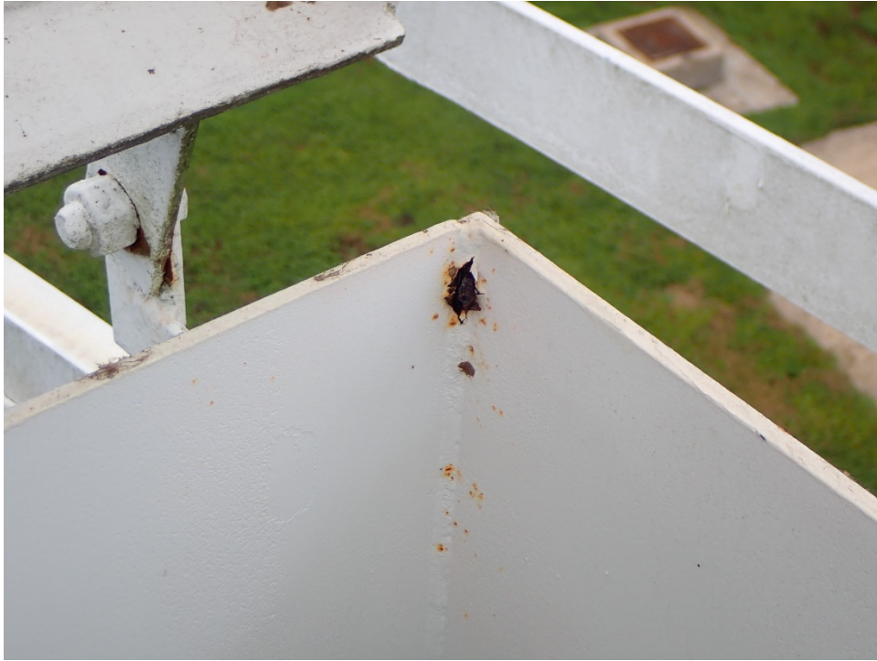
Photo 13: Access hatch with corrosion
