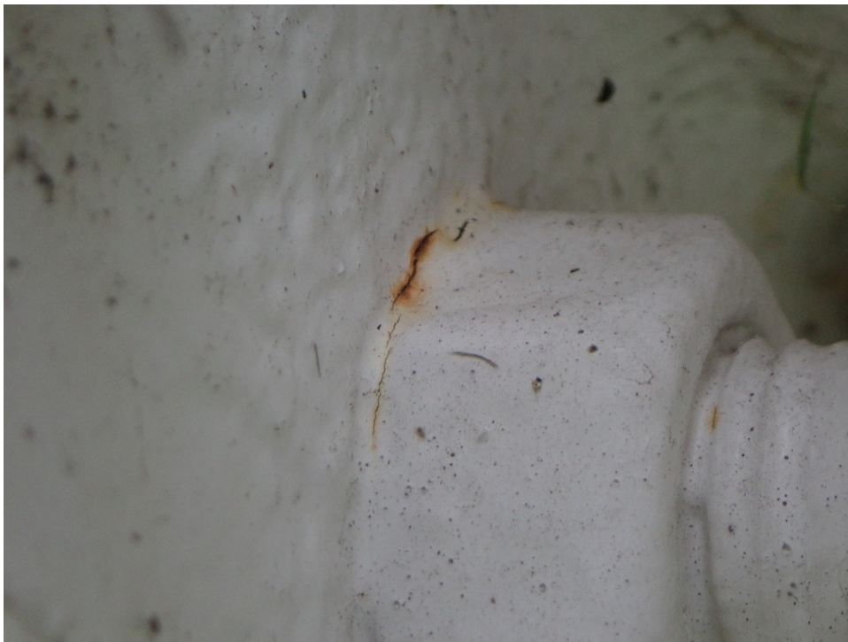
Photo 6: Suction line hardware with corrosion
