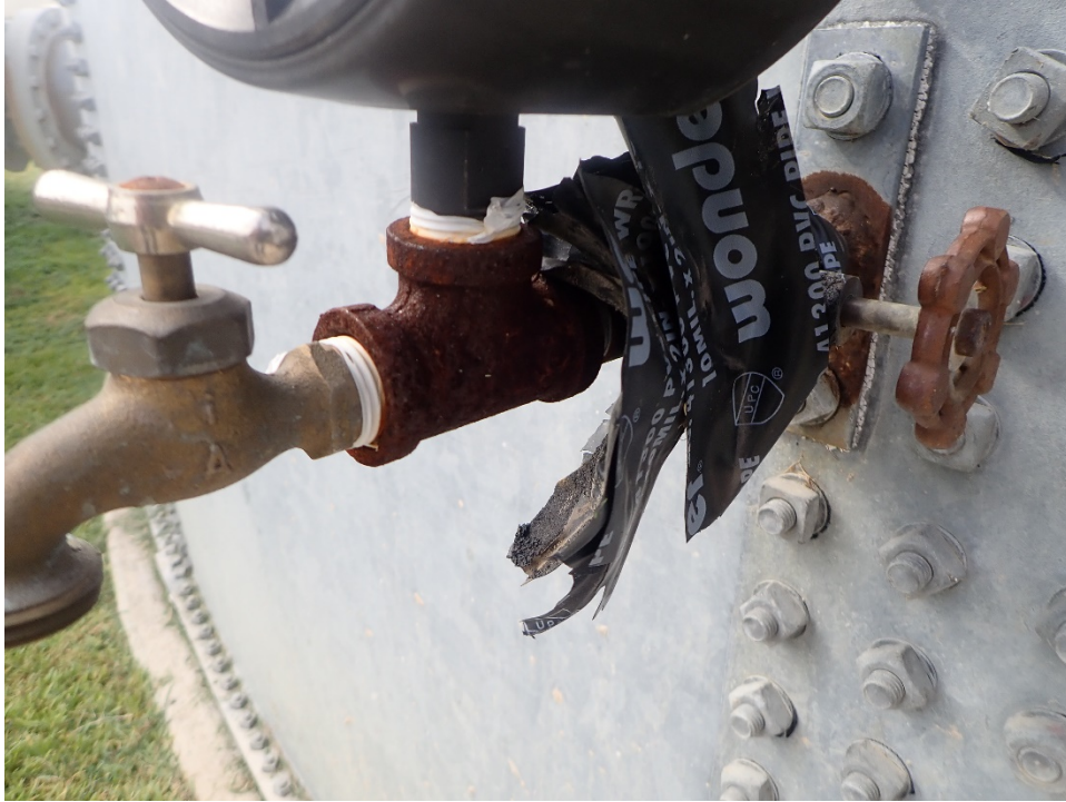
Photo 1: Wall tap with corrosion
