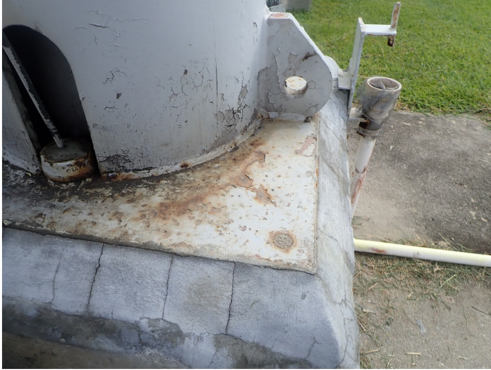
Photo 9: Well piping with corrosion
