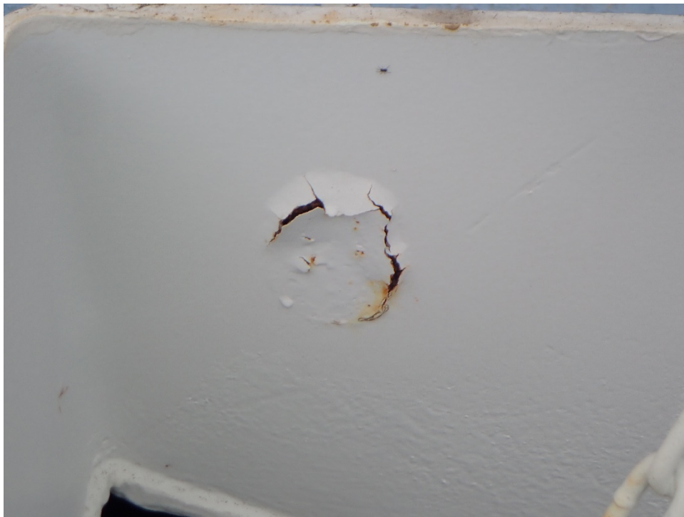
Photo 12: Access hatch with corrosion
