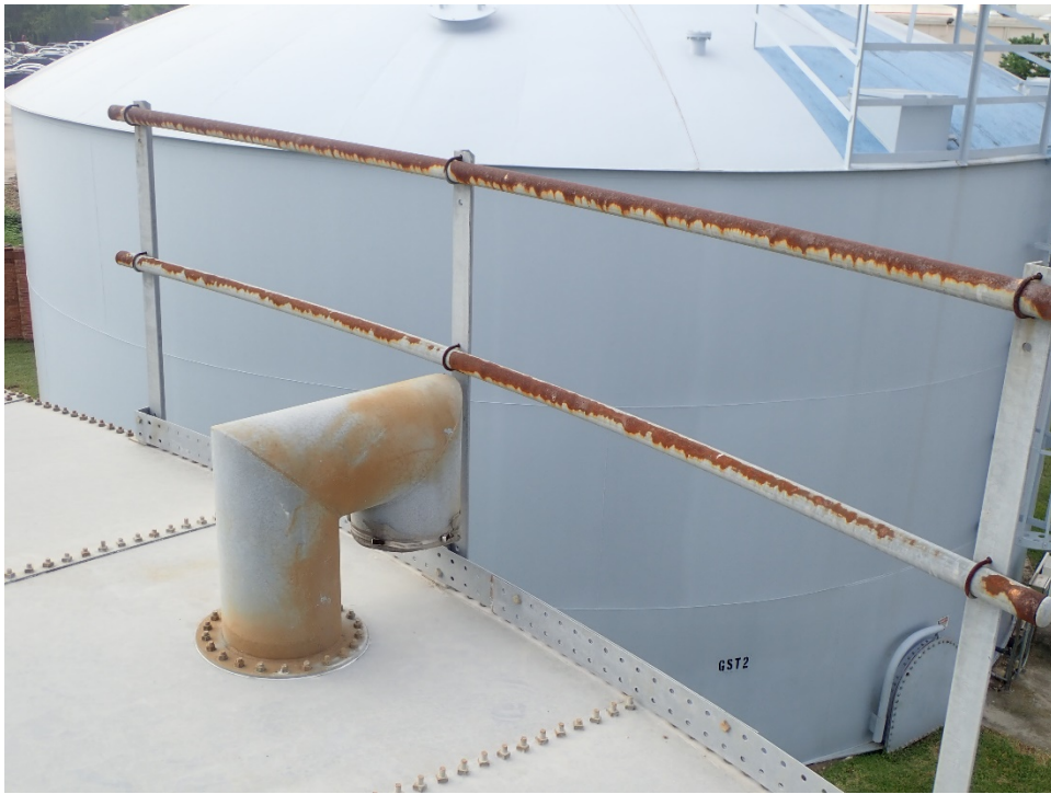
Photo 14: Vent and handrails with corrosion
