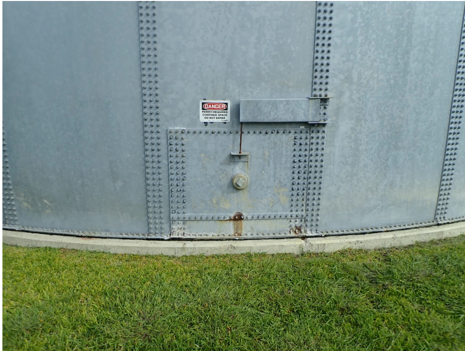
Photo 5: Side hatch with corrosion
