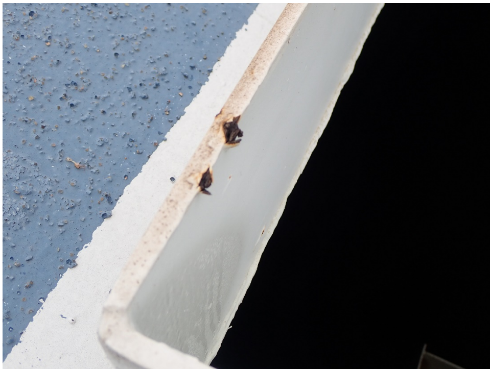
Photo 10: Inspection hatch with corrosion
