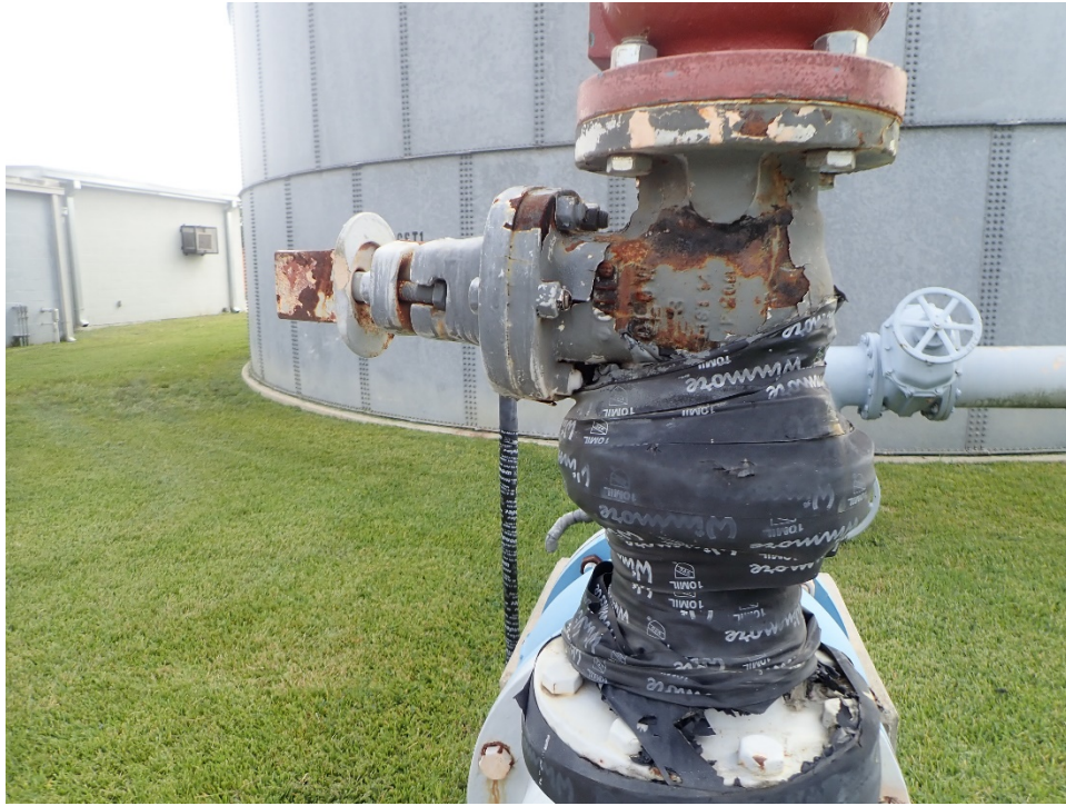
Photo 11: Piping with corrosion
