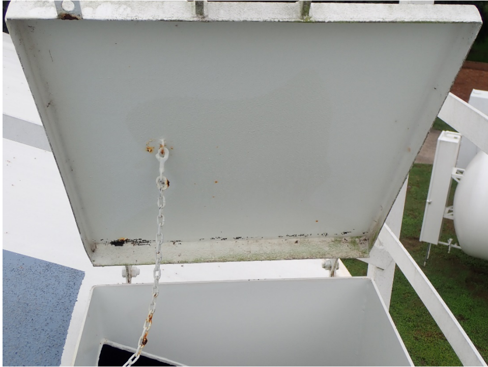
Photo 11: Inspection hatch with corrosion
