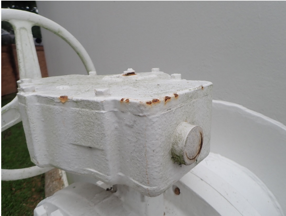
Photo 5: Suction line valve with corrosion
