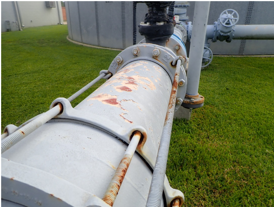
Photo 10: Piping with corrosion
