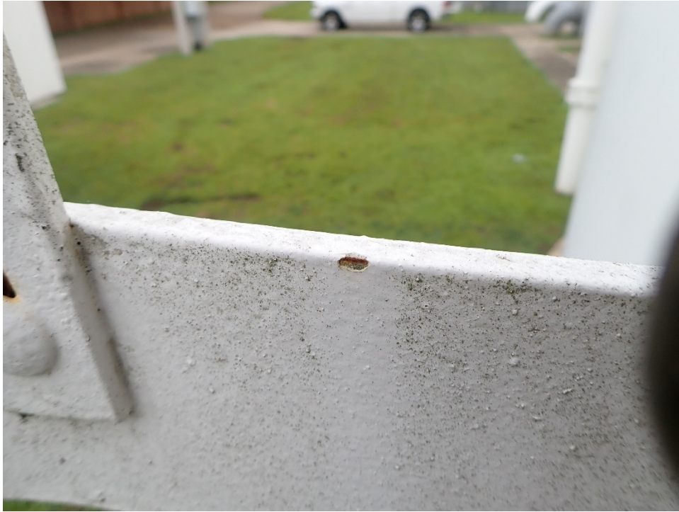
Photo 7: Ladder with corrosion
