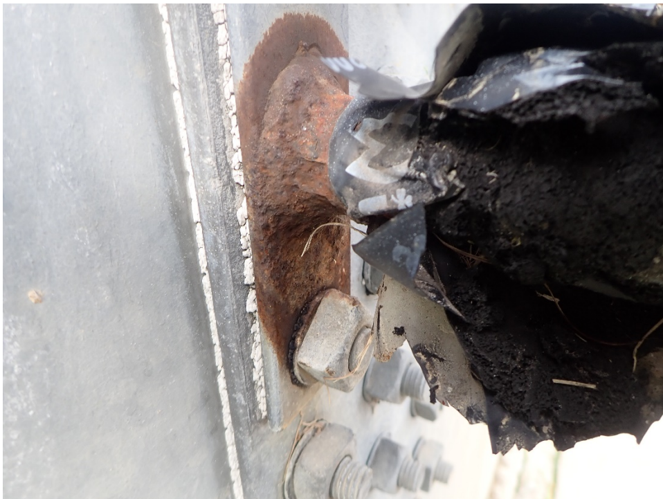
Photo 2: Wall tap with corrosion
