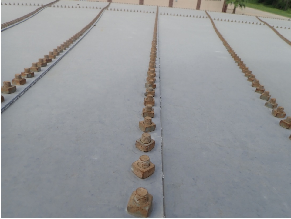
Photo 13: Roof hardware with corrosion
