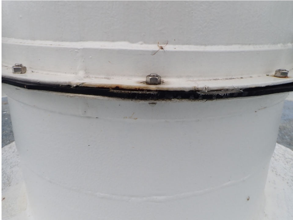
Photo 9: Roof vent with corrosion
