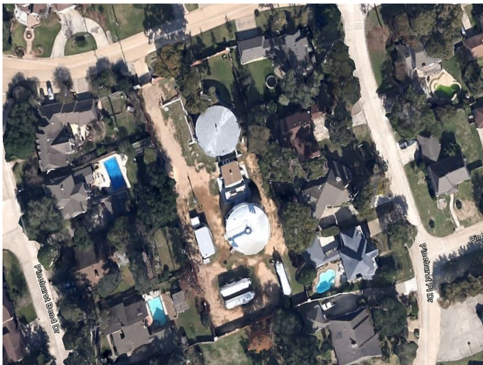
Water plant site overall
