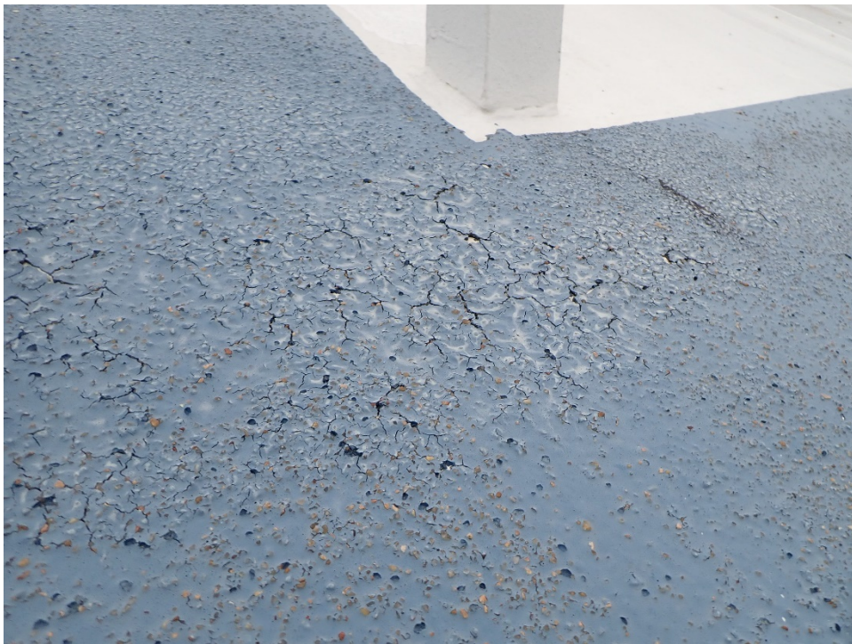
Photo 8: Non-skid coating on roof with coating failure
