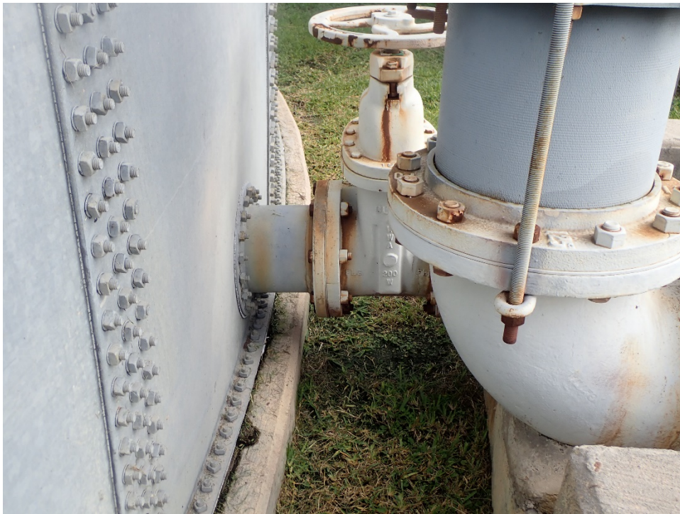
Photo 8: Overflow and drain line with corrosion
