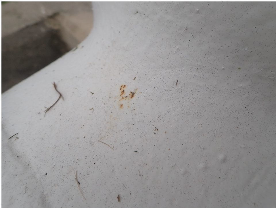
Photo 4: Drain line with corrosion
