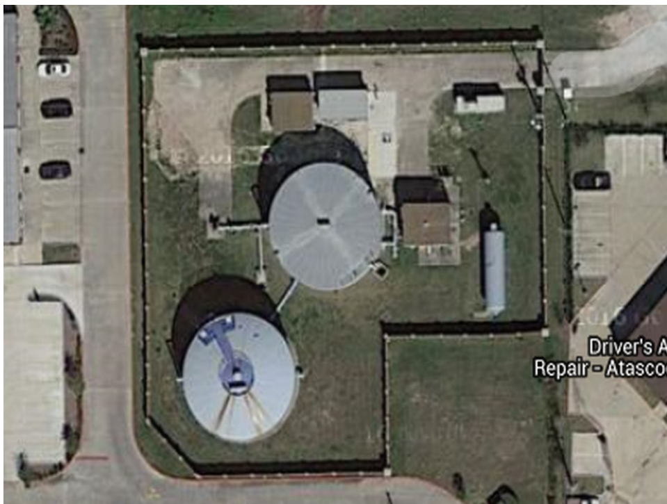
Water plant site overall
