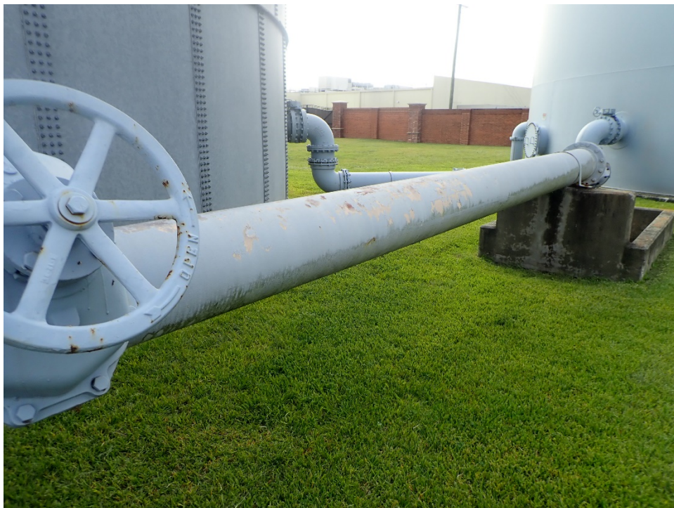
Photo 6: Piping with coating failure and corrosion
