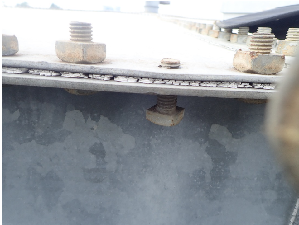
Photo 12: Roof with missing hardware
