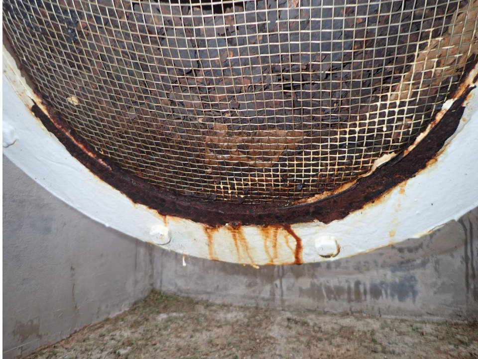
Photo 3: Drain line with corrosion and debris build-up
