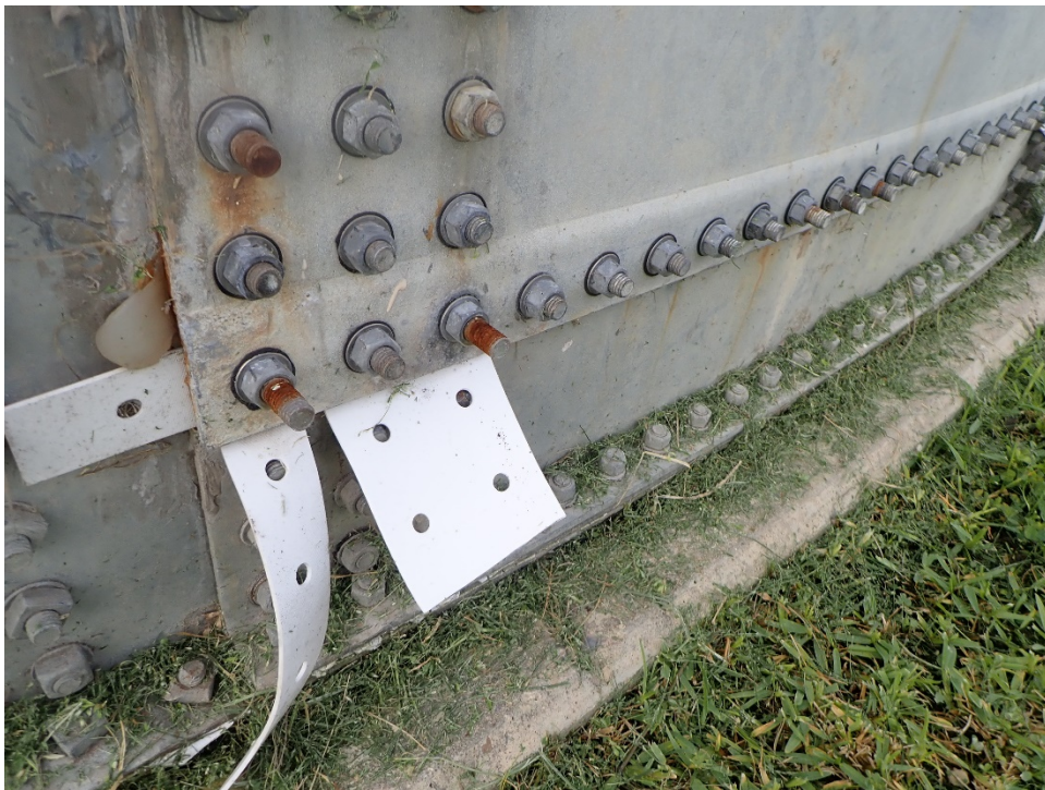
Photo 4: Side hatch with corrosion
