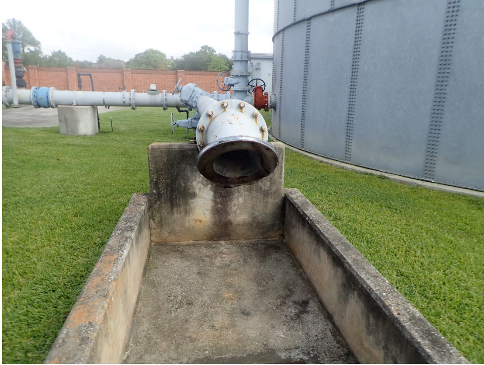
Photo 7: Piping with corrosion
