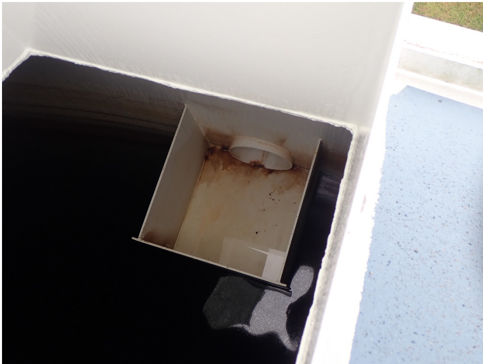
Photo 14: Overflow weir with corrosion
