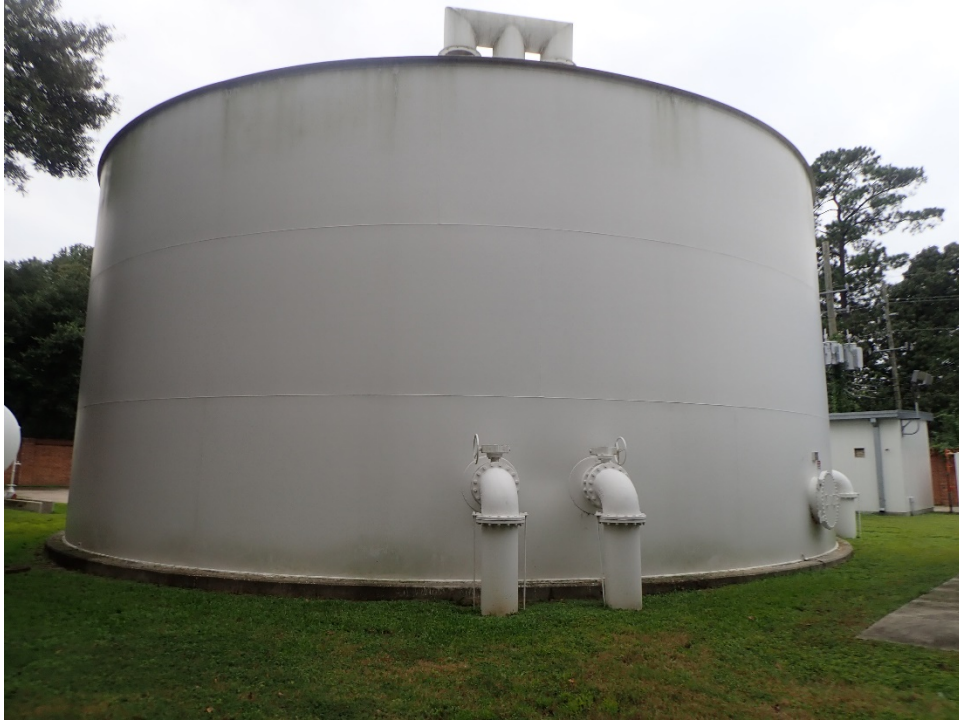
Photo 1: Tank with staining
